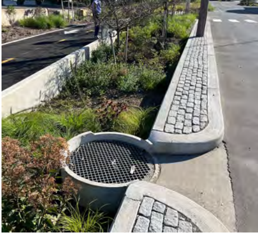
Runoff enters chamber via curb-cut and inlet apron
