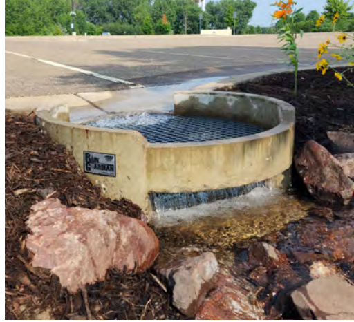
Provides stable inlet and effective pretreatment
